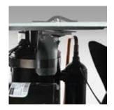
Compressor is bracketed at top as well as bottom to minimize vibration and movement while under way.
